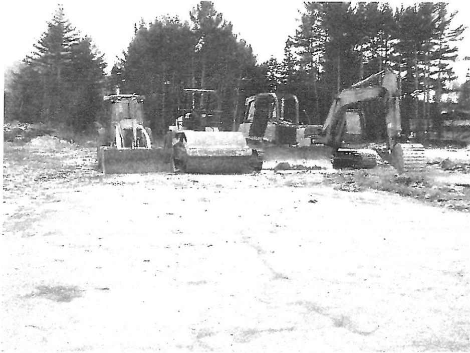
Photo 7: Construction equipment staging behind remaining portion of old motel.
